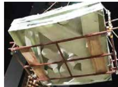
5 Completed panels — with finished A surface (top) and B surface (bottom) — were demolded and shipped to the MOTF site for installation.
