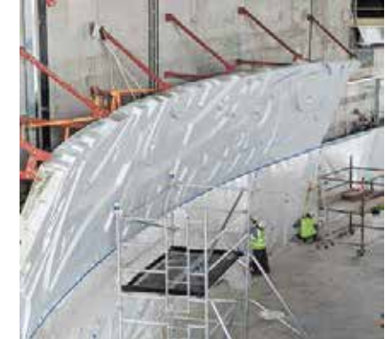
6 Finished panels were bolted to each other and to the steel brackets attached to the building structure.
