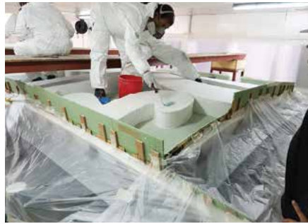
3 CNC-cut EPS foam supports were bonded onto the cured A surface laminate and coated with a light GFRP laminate.
